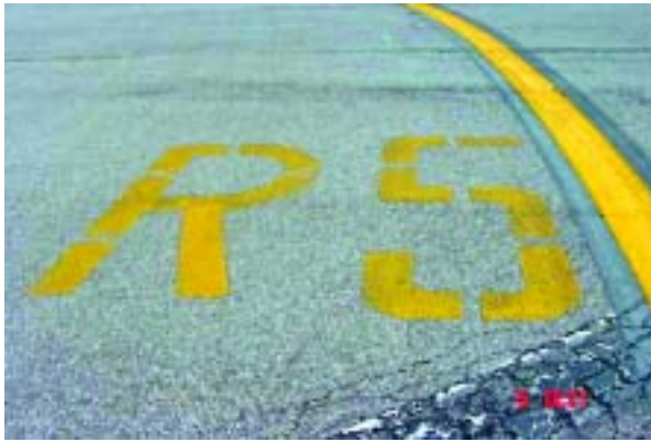
Photograph 6 Marking showing direction TWY R5.
