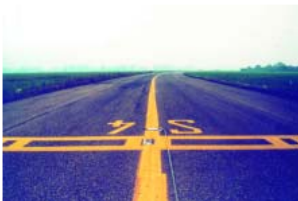
Photograph 9 - S4 marking and ICAO pattern B runway - holding.
