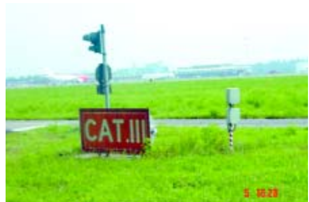
Photograph 13 – CAT III vertical sign on TWY R6.
