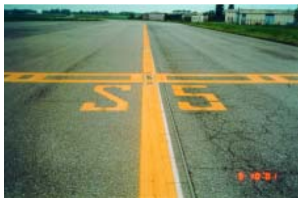
Photograph 10 - S5 marking and ICAO pattern B runway - holding.
